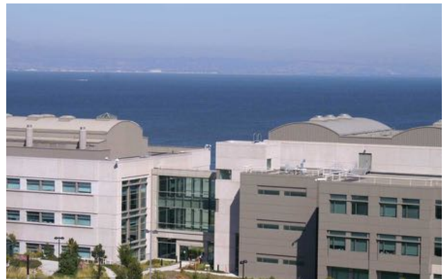
Rooftop screens camouflage building equipment in FRC from views in Upper Campus.
