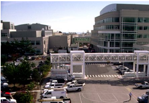
Utility structure within Lower Campus reflects the use of bridges along the Central Spine.
