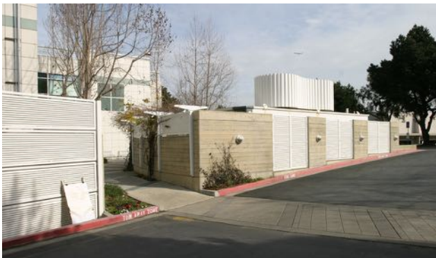
Existing utility enclosure using materials that blend with surrounding architecture.
