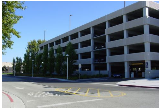
Existing Lower Campus parking structure with landscape buffer along façade.
