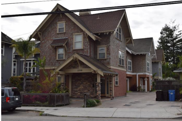
Third floor of living area built into pitched roof element to reduce appearance of height.
