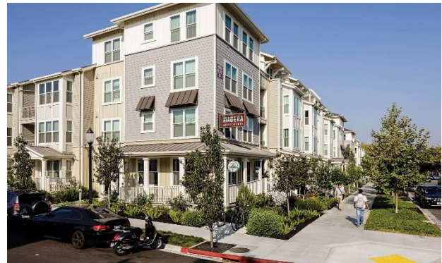
Variation in building heights, facade articulation, landscaped setback, and street trees.
