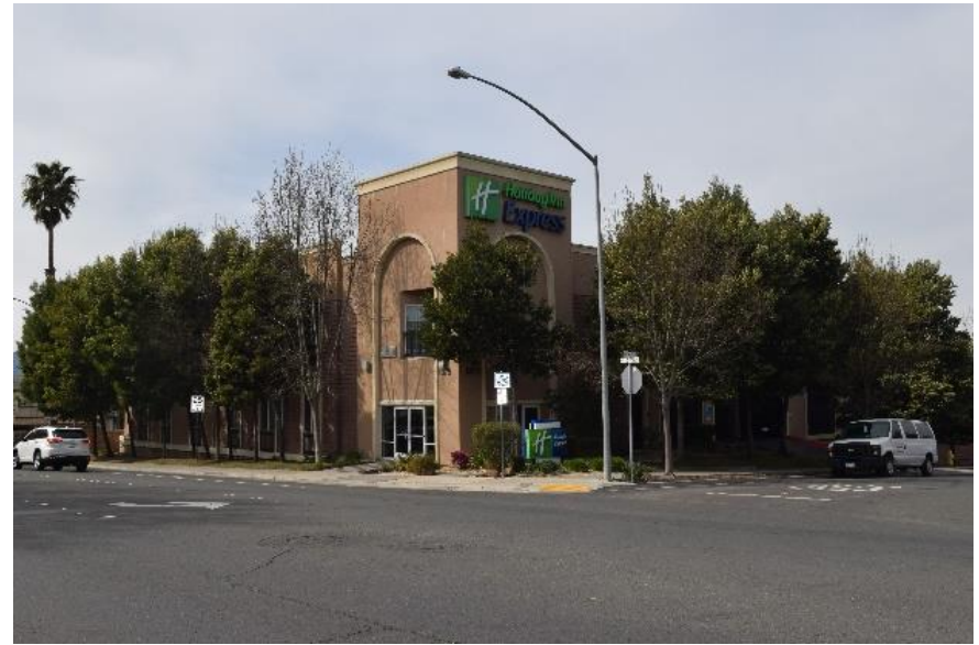
Holiday Inn: 39 ft. at corner element and 32 ft. adjacent building wall
