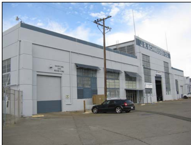
Benicia Arsenal Machine Shop (Building 91), built in 1942 and enlarged in 1951. (Source: Page & Turnbull, May 2010)
