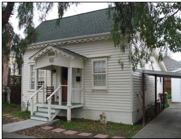
149 East D Street, 1854. Although the trim work may be a replacement, it is in keeping with Gothic Revival ornamentation of the period. (Source: Page & Turnbull, January 2010)
