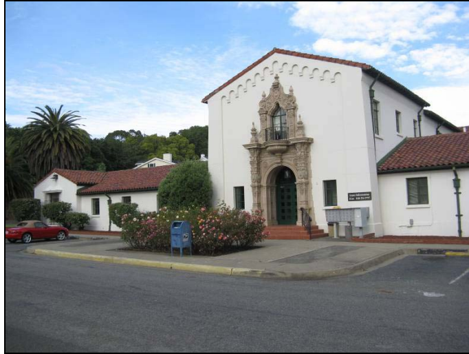
Main Headquarters (Building 92), 1942. This ornate building stands in stark contrast to the more utilitarian structures built during World War II. (Source: Page & Turnbull, May 2010)
