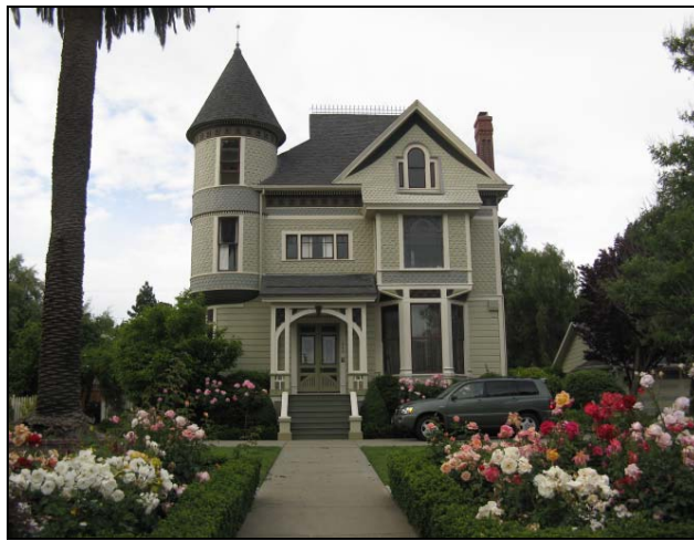
The Riddell-Fish House at 245 West K Street, 1888. This is Benicia’s finest Queen Anne residence and a city landmark. (Source: Page & Turnbull, May 2010).
