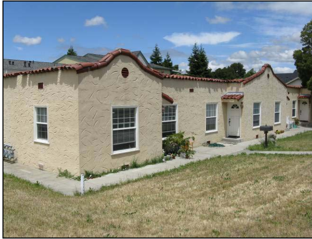
801 – 807 East H Street, circa 1930s. This triplex is a somewhat rare example of multi-family housing in this style. (Source: Page & Turnbull, May 2010)
