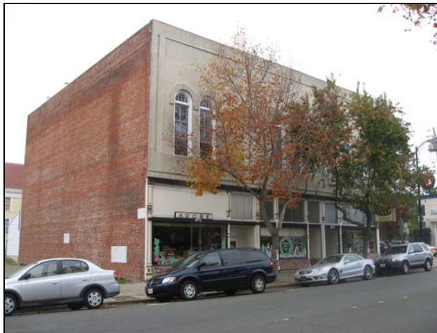
New Masonic Lodge at 935 First Street, built in 1890. An elaborate cornice and beltcourse has been removed, but most of the storefronts are intact. (Source: Page & Turnbull, January, 2010)
