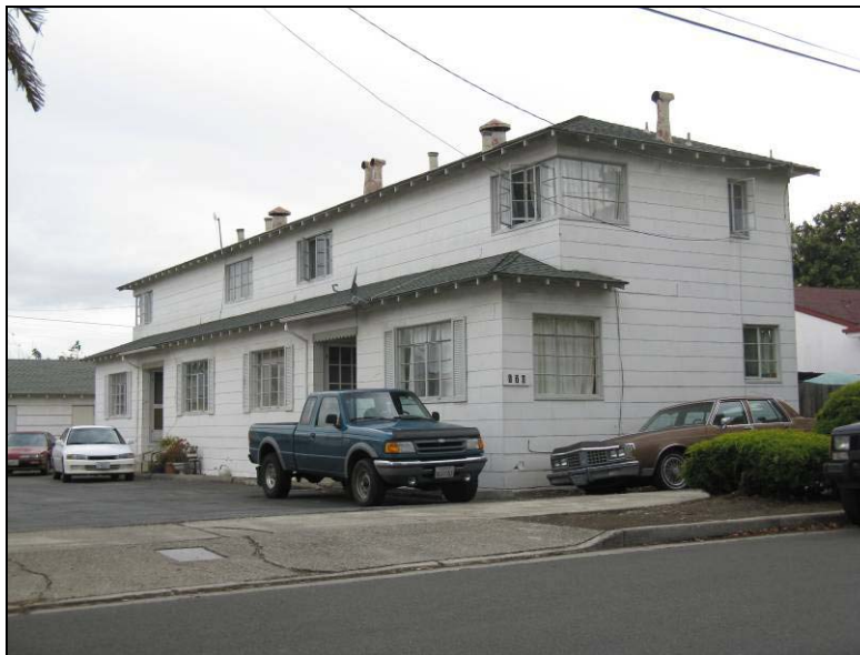
170 West K Street. This design is very typical of public housing constructed during World War II. It has been re clad with asbestos shingles, but the windows appear to be original. (Source: Page & Turnbull, May 2010)
