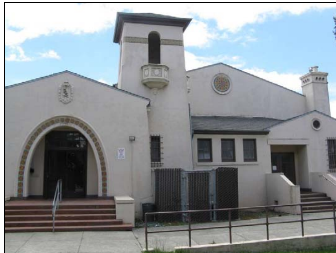
Benicia Grammar School, constructed in 1938 at 350 East K Street. Designed in the Spanish Colonial Revival style, it now houses the Benicia Unified School District Office. (Source: Page & Turnbull, May, 2010)
