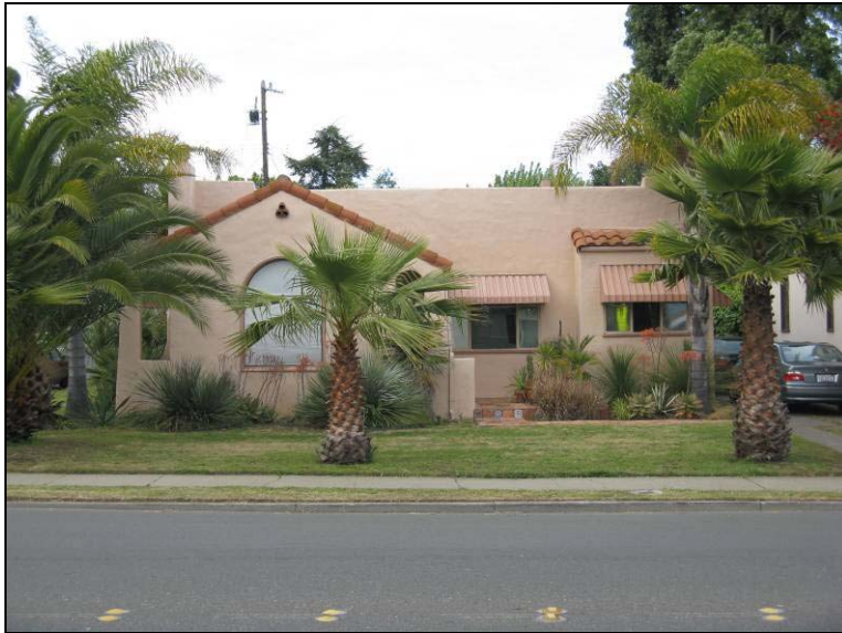
245 Military East, a Spanish Colonial Revival residence constructed in 1930. (Source: Page & Turnbull, May, 2010)
