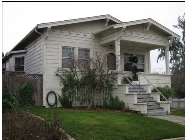
192 West H Street, circa 1910. An early and exceptionally well preserved Craftsman cottage. Note the divided upper window sashes—a very common feature of Craftsman houses. (Source: Page & Turnbull, January 2010).
