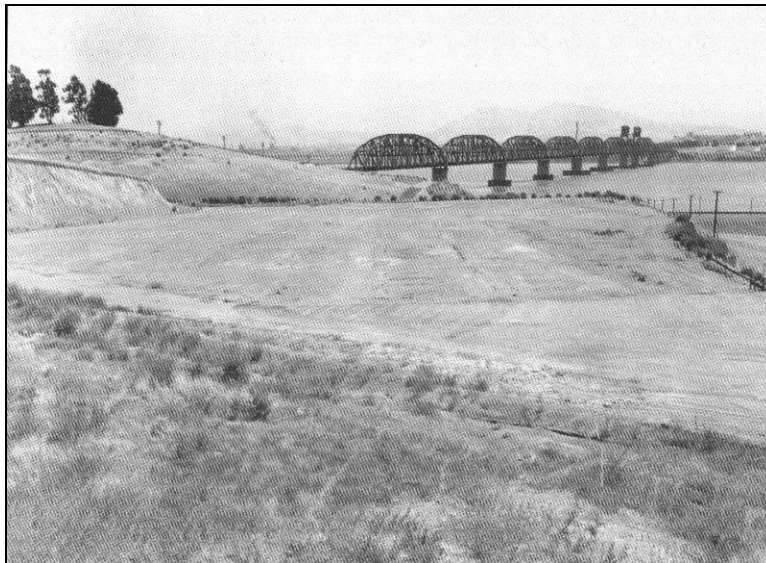
Southern Pacific Railroad Bridge between Army Point and Martinez, n.d. (Source: Benicia Historical Museum)
