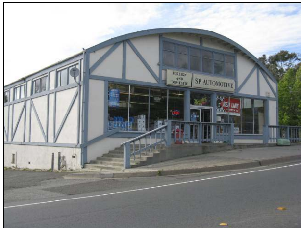
1421 East Fifth, circa 1950. The building's design and massing is more typical of industrial buildings, but the storefront configuration appears original. (Source: Page & Turnbull, May 2010)
