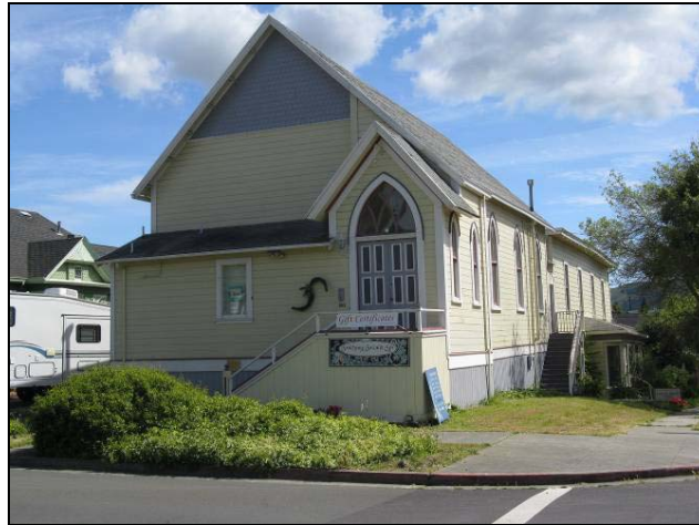
Methodist Church at 190 West J Street (1882). A corner tower has been removed and an addition made to the primary facade, but it still retains most of its original arched windows. (Source: Page & Turnbull, May, 2010)
