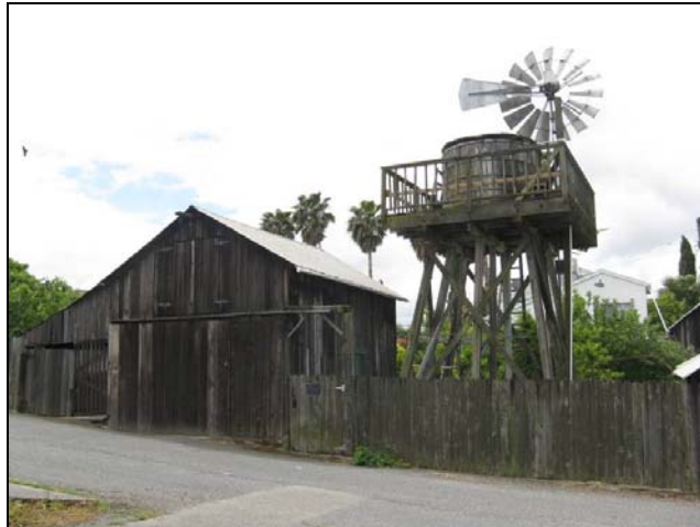
Horse stable, windmill and water storage tank located behind 553 East G Street. Note the block and tackle arm beneath the gable end of the stable. (Source: Page & Turnbull, May 2010).
