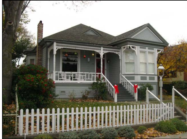
121 West J Street, circa 1905. This form was very popular around the turn of the century. (Source: Page & Turnbull, January 2010).
