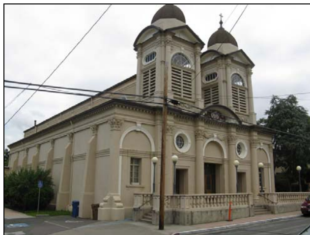
St. Dominic's Church at 475 East I Street. (Source: Page & Turnbull, May 2010)
