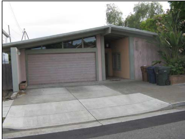
The former Benicia Public Library at 144 East G Street, now converted to a private residence. (Source: Page & Turnbull, May 2010)
