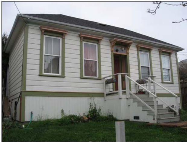
175 East F Street, circa 1880. A very modest example of an Italianate cottage. While the windows and doors have been replaced, it retains its fenestration pattern and window hoods. (Source: Page & Turnbull, January 2010).
