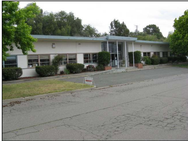
675 East H Street, circa 1950. This International style building was constructed for Yuba Manufacturing. Today it houses a glass works. (Source: Page & Turnbull, May 2010)
