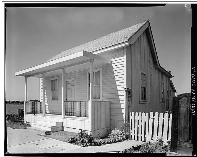
145 West D Street, circa 1850. This “saltbox” style house shows the simple construction methods that characterized much of Benicia’s earliest residences. (Source: Library of Congress, 1977 HABS photograph CAL, 48-BENI, 5-15).
