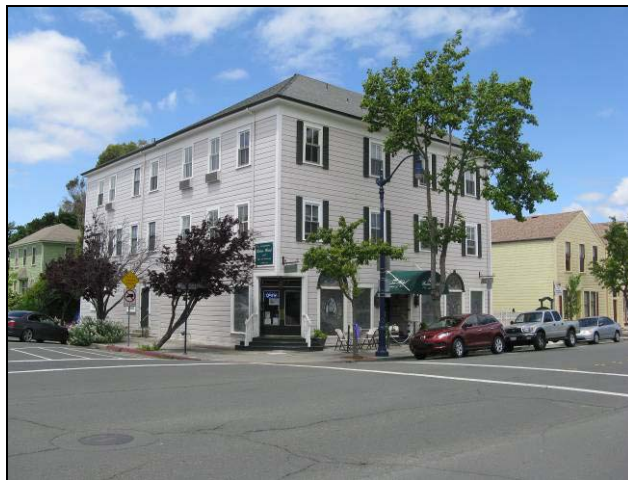
The Union Hotel at 401 First Street, built circa 1860. Investigations show the building originally included a cantilevered porch above the first story. (Source: Page & Turnbull, May 2010)
