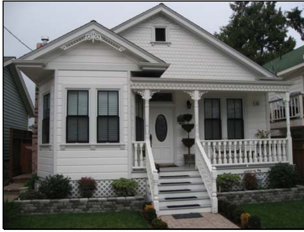
185 East D Street, circa 1900. A good example of a Queen Anne cottage. Note the scrolled brackets on the porch and fish scale shingles in the gable end. (Source: Page & Turnbull, January 2010)
