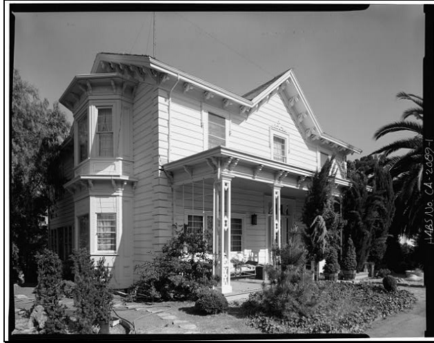
Bishop Wingfield's House, constructed ca. 1875. The bay window, quoins and brackets are Italianate in style, but the sharply peaked roofline is a holdover from Gothic Revival designs. (Source: Library of Congress, 1976 HABS documentation)
