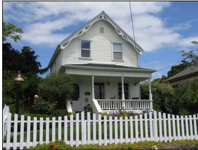
351 East K Street, circa 1870. The elaborate verge boards show clear Gothic Revival influence. (Source: Page & Turnbull, May 2010)
