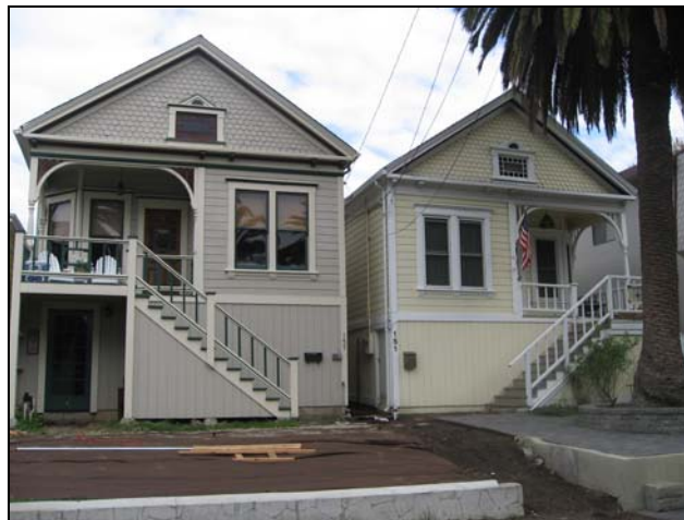
151 & 155 West J Street, circa 1895. Originally constructed as mirrored Queen Anne cottages, the building at left has been raised to insert a basement apartment. (Source: Page & Turnbull, January 2010).
