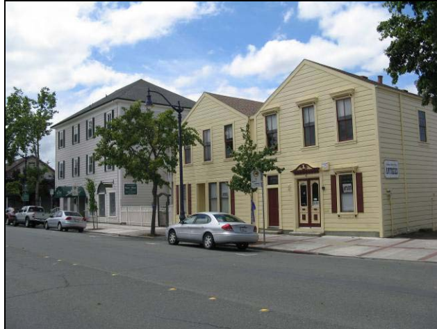
The City Hotel at 415 First Street, circa 1860. The building was cut in half for moving, and the pieces assembled alongside one another. (Source: Page & Turnbull, May 2010)
