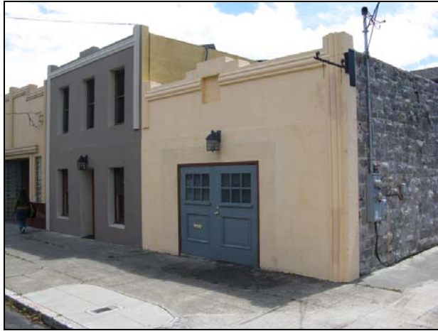
120 – 128 West H Street. The two buildings at right appear to have been connected with the Benicia Brewery. They have been altered with stucco cladding and Streamline Moderne influenced ornamentation. (Source: Page & Turnbull, May 2010)
