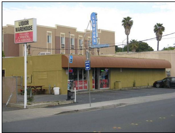
457 Military East, circa 1950s. Several windows on this building appear infilled, but it likely retains its original neon sign. (Source: Page & Turnbull, May 2010)
