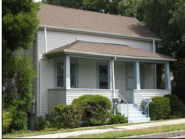
535 East G Street, circa 1860s. The Craftsman porch and windows are later additions, but the building's massing is indicative of its early construction. (Source: Page & Turnbull, May 2010)
