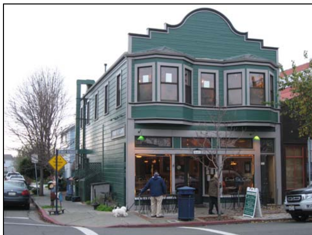
440 First Street. The bay windows were likely not added until circa 1915. (Source: Page & Turnbull, January 2010)
