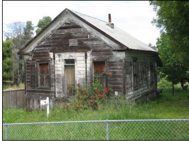
551 East H Street, circa 1860. Though badly neglected, this building appears to retain its original door. The outline of the former porch is also visible. (Source: Page & Turnbull, May 2010)
