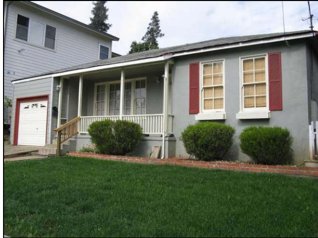
22 Buena Vista Street, 1943. Though clad in replacement stucco, the windows of this house appear original. (Source: Page & Turnbull, May 2010)
