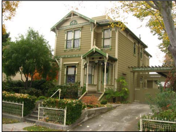
140 West I Street, circa late 1880s. A particularly strong example of the Stick/Eastlake style. Note the decorative truss in the gable end and extended brackets. (Source: Page & Turnbull, January 2010).
