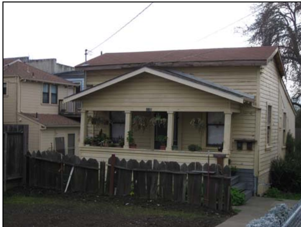
110 West G Street, circa 1855. The Craftsman-style porch is likely a later construction. Note also the small rear addition. (Source: Page & Turnbull, January 2010).
