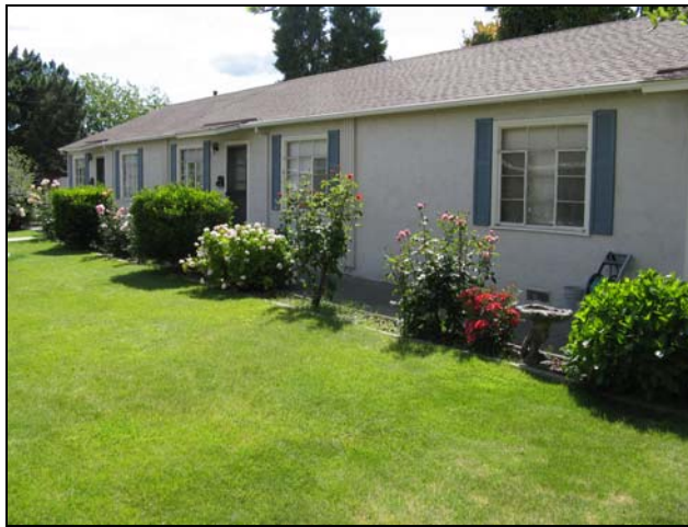
170 West J Street, ca. 1940s. This is one of two mirrored triplexes, and was likely used for multi-family housing during World War II. (Source: Page & Turnbull, May 2010)
