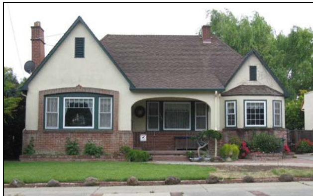
130 West K Street, 1928. This building is identical in design to 261 Military East and likely designed by the same architect/builder. (Source: Page & Turnbull, May 2010)
