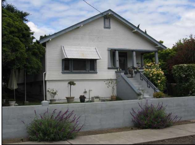
451 East H Street, circa 1915. Note the wood bevel siding. (Source: Page & Turnbull, May 2010)
