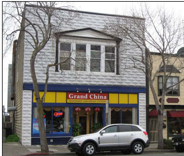
718 First Street, constructed circa 1905 – 1910. Based on historic photographs, the unusual false brick cladding appears original, as does the upper window with its pediment.. (Source: Page & Turnbull, May 2010.)
