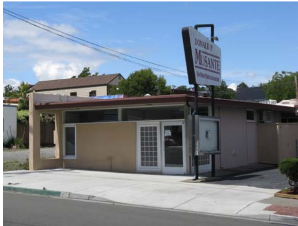
127 East H Street, circa 1955. This buildings shows strong International Style influence. The sign is original. (Source: Page & Turnbull, May 2010)
