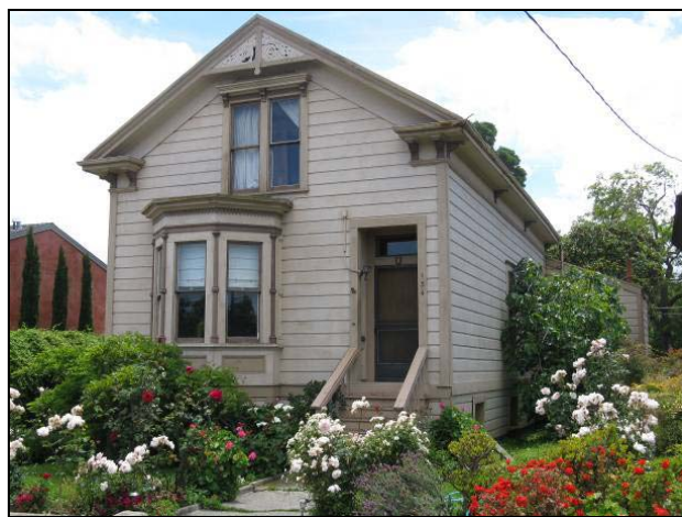
134 West H Street, circa 1880. The gable returns are usually indicative of the Greek Revival Style. But the slanted bay window with colonettes, roof brackets and attic window hood are more indicative of Italianate influence. (Source: Page & Turnbull, May 2010)
