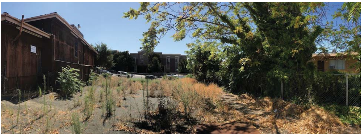
Building Exterior/Parking Lot Area View Facing N Street
