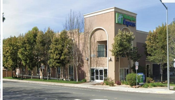
Holiday Inn Express, 1375 Fifth Street 39 ft. at corner element; 32 ft. adjacent building wall
